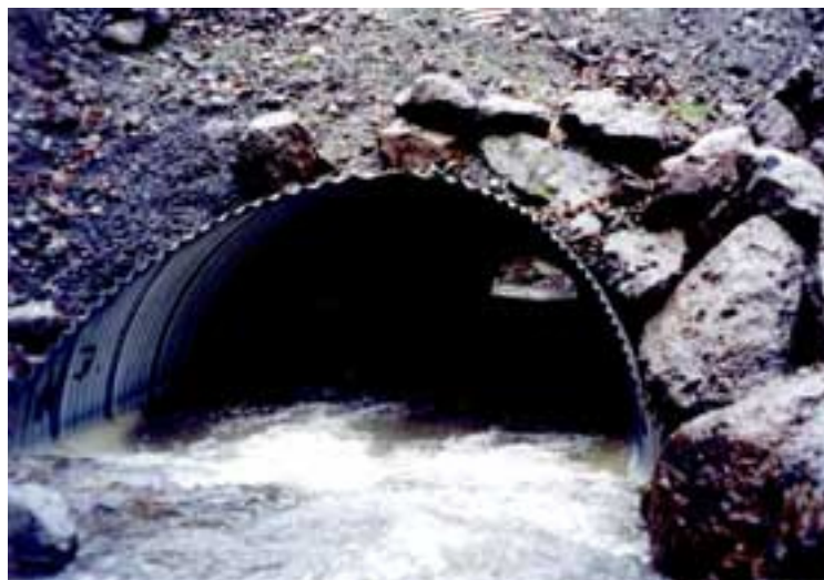
Culvert inlet, "daylight" riser noticeable in the upper center of photo
