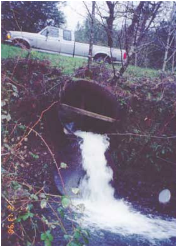
Outlet before replacement, 02/13/98
