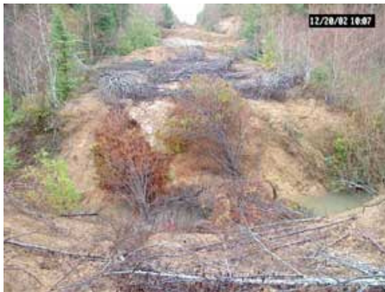
Looking from the south at the excavated channel and placed trees, 12/20/02
