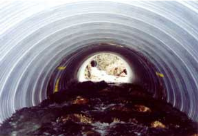
Looking upstream through the culvert at boulders
