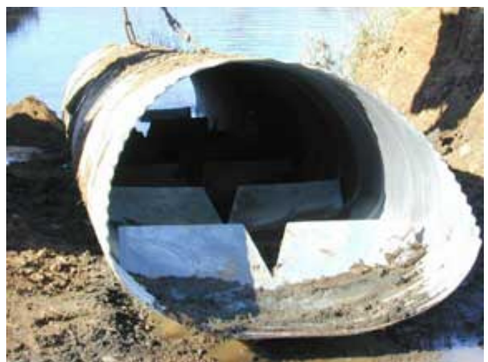
Looking upstream into the baffled culvert during installation, 2002
