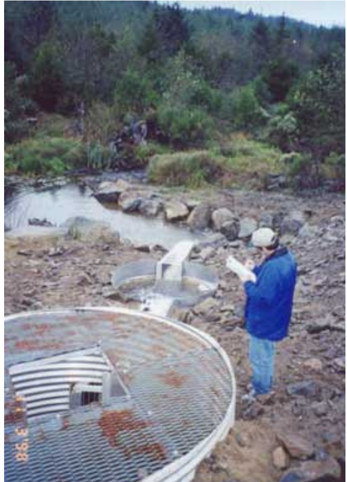
Looking downstream at resting risers and chutes, 11/03/98
