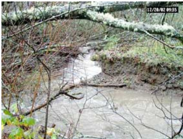
Looking upstream at split channel - terminus of the headcut migration from culvert removal, 12/20/02
