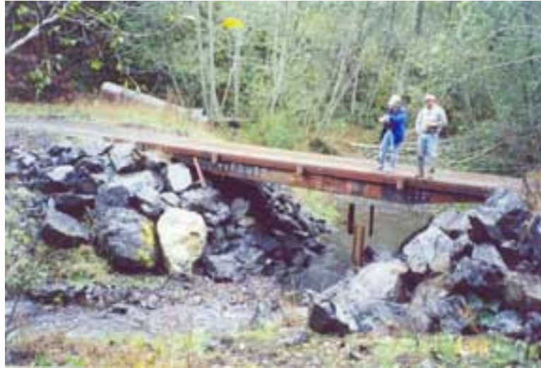
Looking downstream at the railcar bridge
