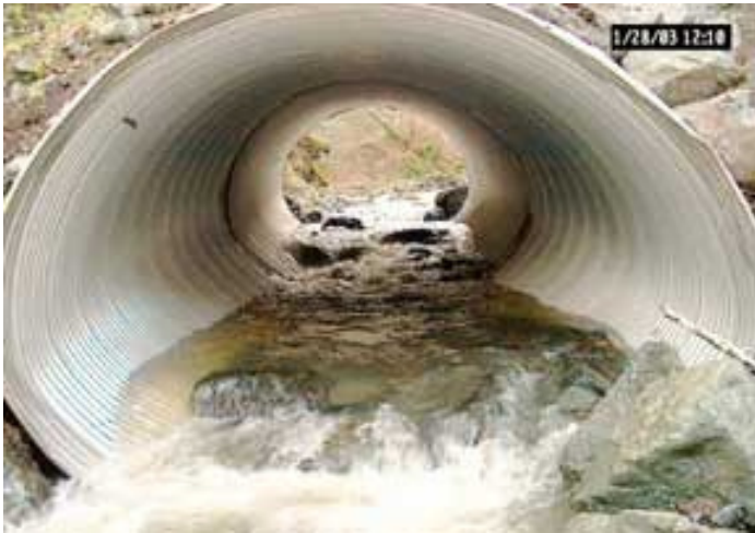
Looking at rip rap forming pools
