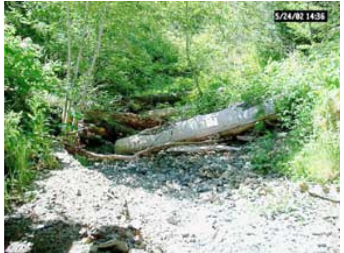
Looking downstream from beneath the bridge at wood placement
