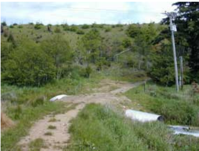
Full view of culvert placed at the downstream reservoir, 5/15/03
