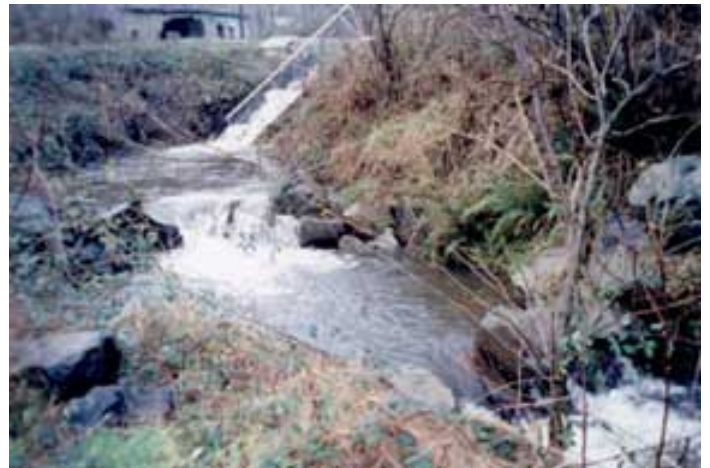
Boulder weir constructed to raise water level at fish ladder upstream, 11/96 View of original weir and first new downstream weir, 01/99
