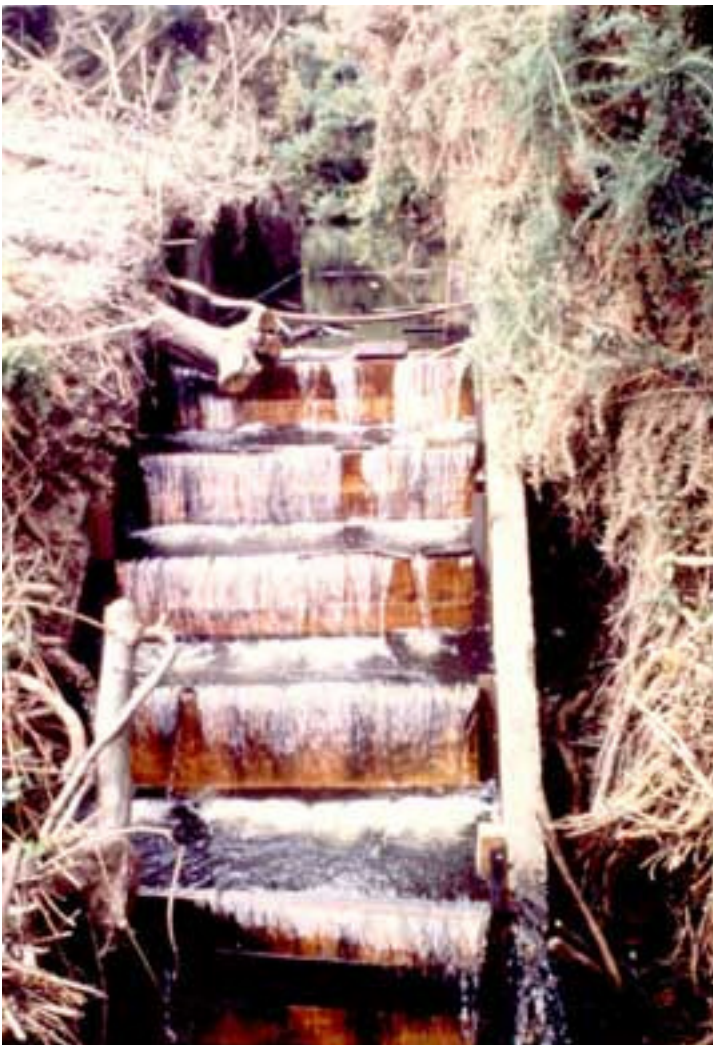
Fish ladder needing maintenance and bottom jump too high, 08/95 New fish ladder with water level raised by boulder weirs, 01/99
