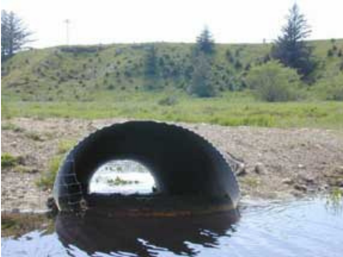
Culvert inlet at the downstream reservoir, 5/15/03
