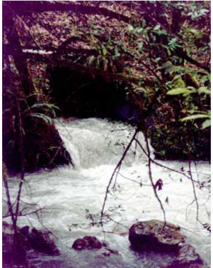
View from road looking downstream at three boulder weir steps Culvert outlet drop with reduced height due to boulder steps
