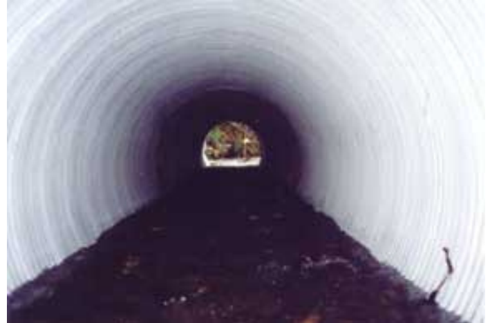
Substrate in culvert, 01/12/00
