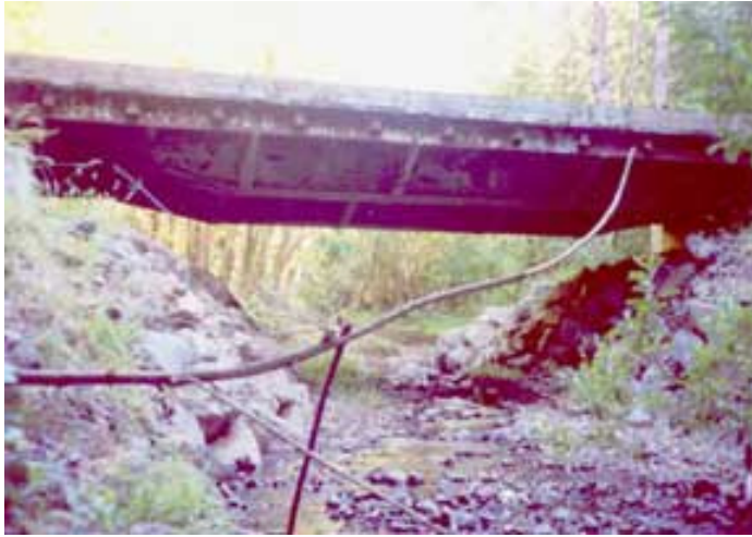
Looking upstream newly formed channel prior to the first winter, 07/31/00
