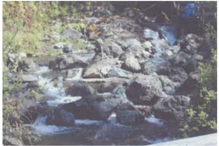
Boulders not performing as weirs, 04/01
