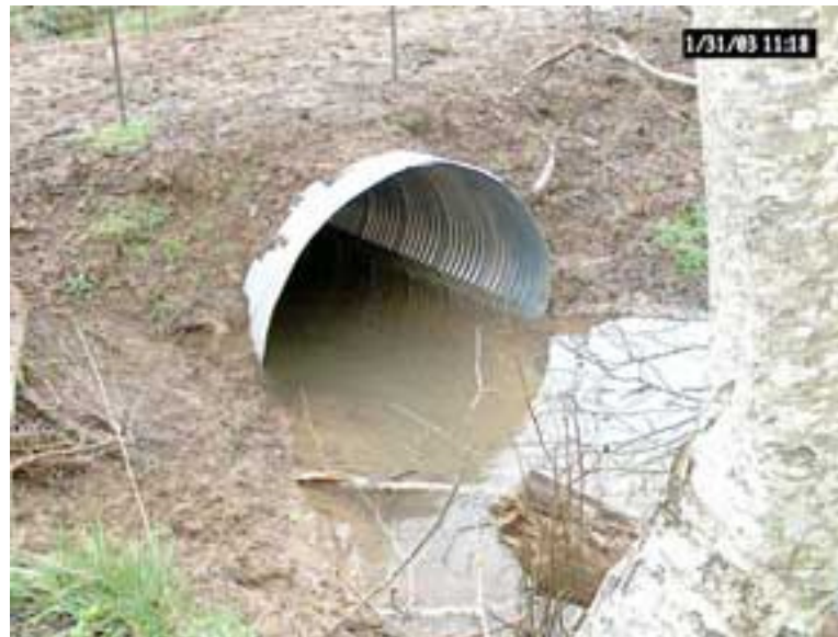
Close-up of outlet following installation, 01/31/03
