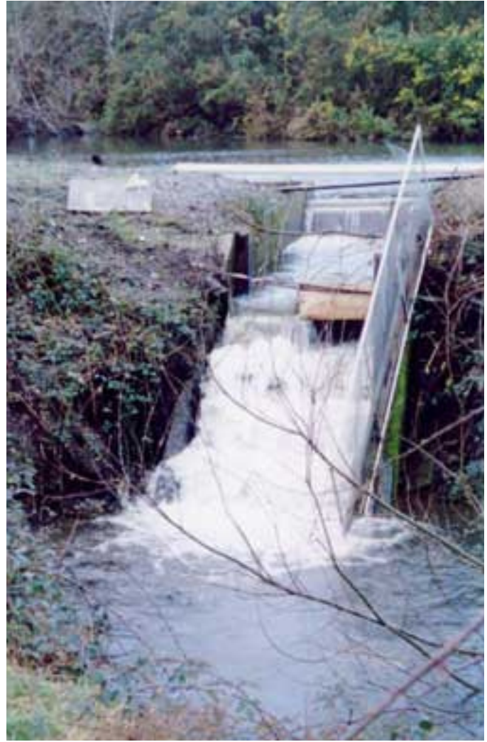
Fish ladder needing maintenance and bottom jump too high, 08/95 New fish ladder with water level raised by boulder weirs, 01/99
