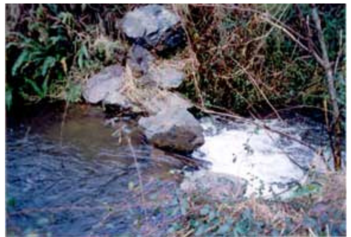
Original boulder weir with smaller step after more weirs installed, 01/99 Closeup of first new downstream weir, 01/99
