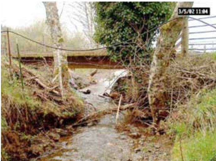
Looking downstream at the bridge placed at the lower crossing, 03/05/02
