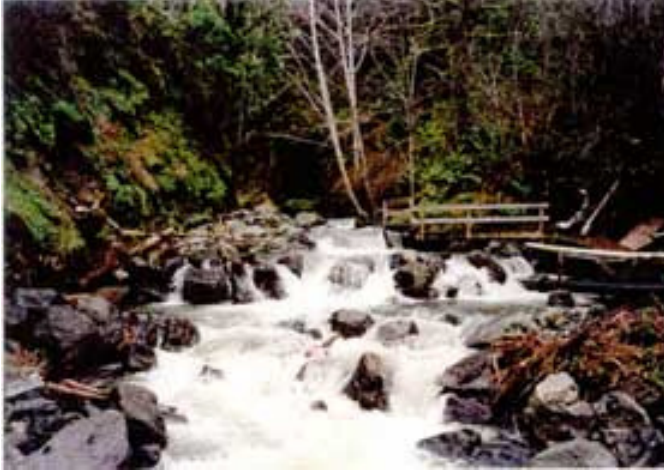
Steps formed by boulder weirs, 03/22/99
