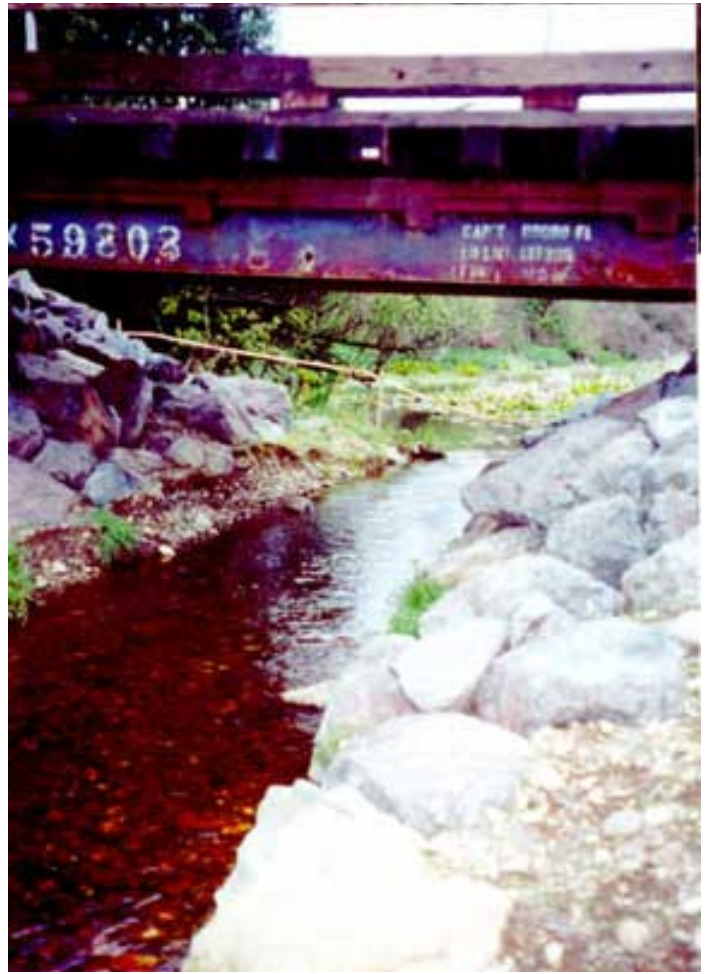
Looking upstream after installation of bridge, 03/15/00
