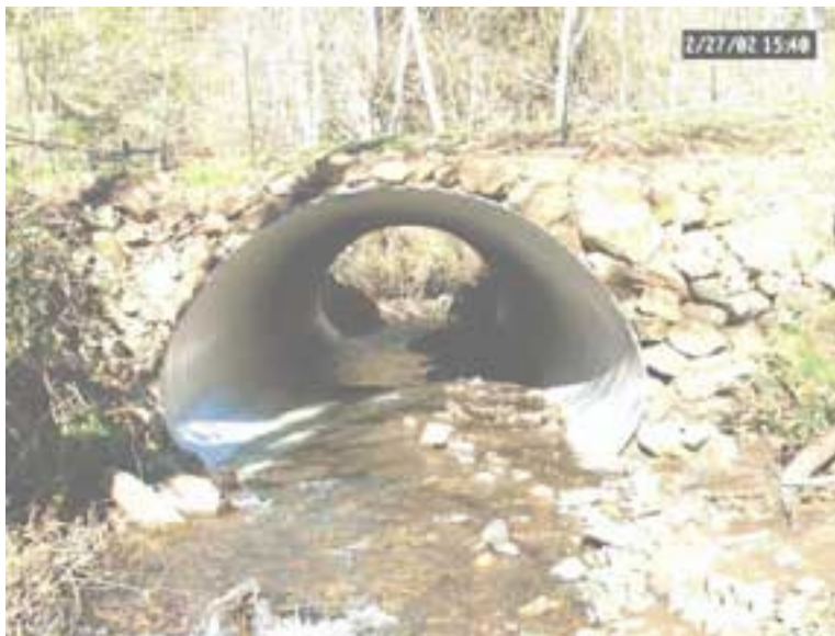
Looking upstream at the countersunk culvert, notice shallow deposition, 02/27/02
