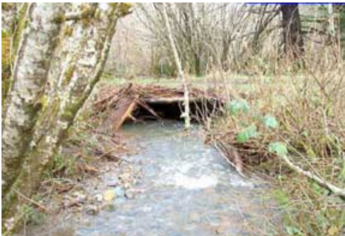
Looking at the former inlet of the upper crossing, 01/28/02
