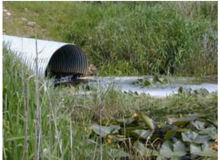
Culvert outlet at the downstream reservoir, 5/15/03
