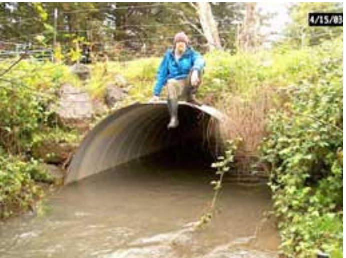
Outlet of the downstream countersunk culvert, 04/15/03
