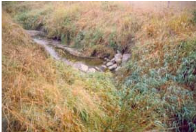
Upstream weir following construction
