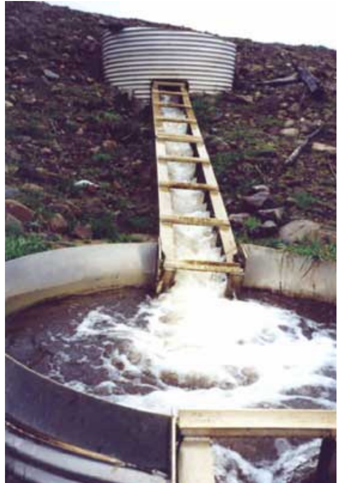
Close-up of flow in resting riser looking upstream, 02/02/99
