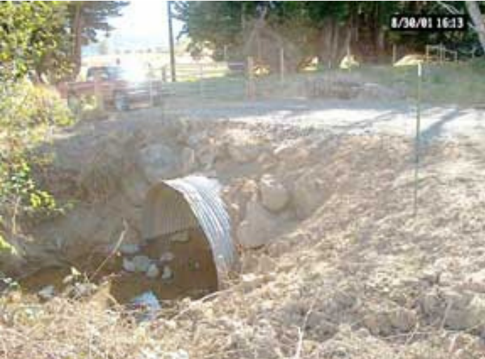
Outlet of the downstream culvert following installation, 08/30/01
