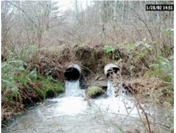
Looking at the former outlet of the lower crossing, 01/28/02
