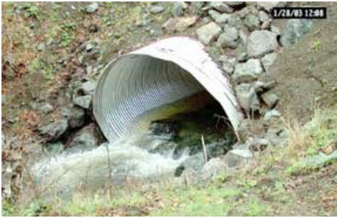
Looking through culvert at inlet knox 1 mp 1.130 Outlet
