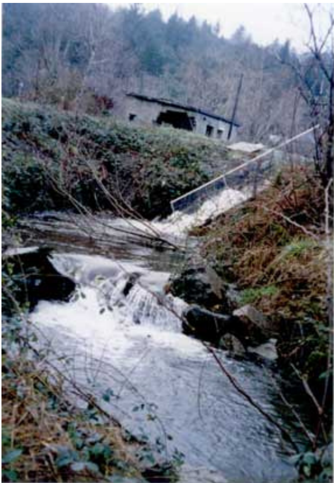
Original boulder weir with smaller step after more weirs installed, 01/99 Closeup of first new downstream weir, 01/99
