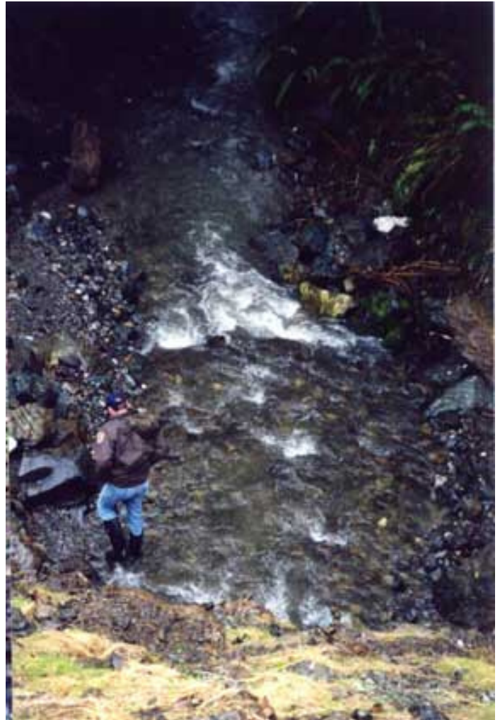
Outlet with jump pool weirs, and straw mulch on road fill
