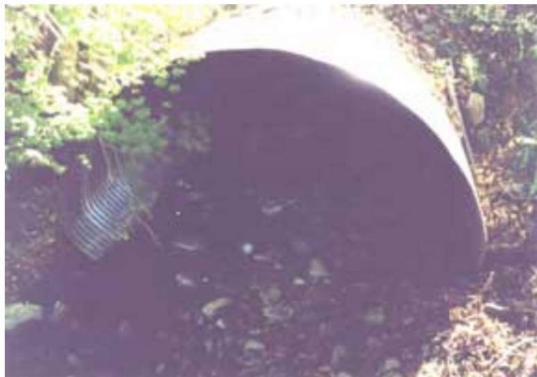
Looking upstream at outlet from riprap
