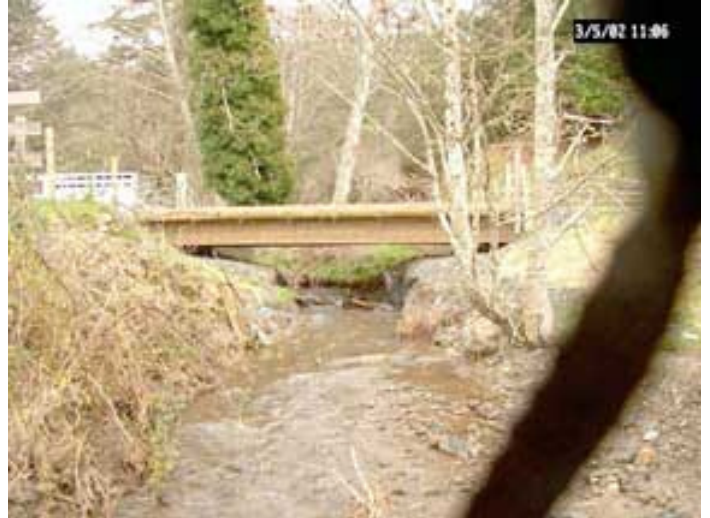
Looking upstream at the bridge placed at the lower crossing, 03/05/02
