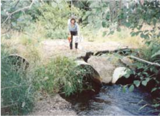
Outlet of former crossing – notice 3 culverts, 2 of which are failing Looking from upstream at the bridge
