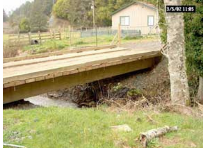
Looking from the SE at the lower crossing bridge, 03/05/02
