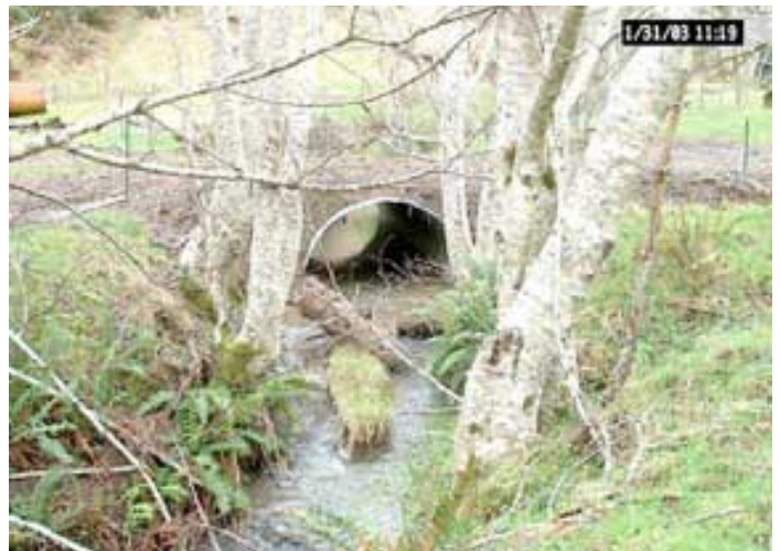
Looking upstream at the outlet following installation, 01/31/03
