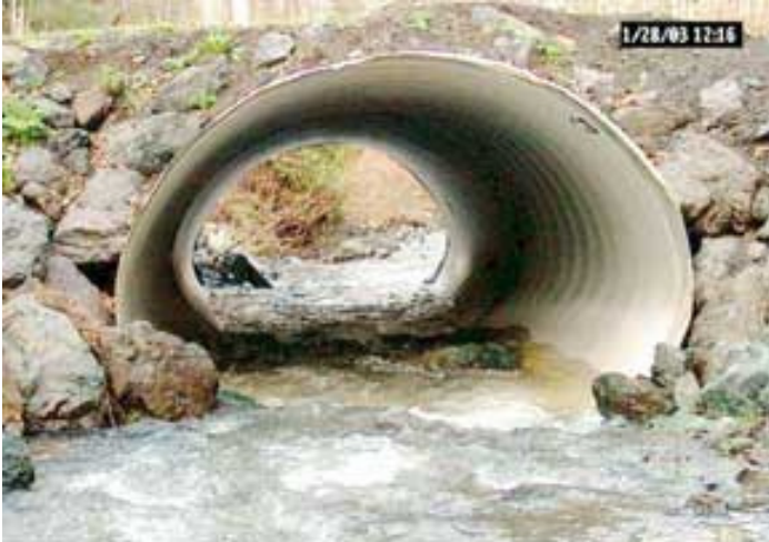
knox1 mp 1.130 Looking at inlet knox 1 mp1.130
