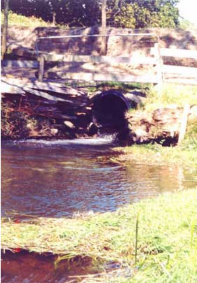
Looking upstream before installation of bridge, 04/23/99
