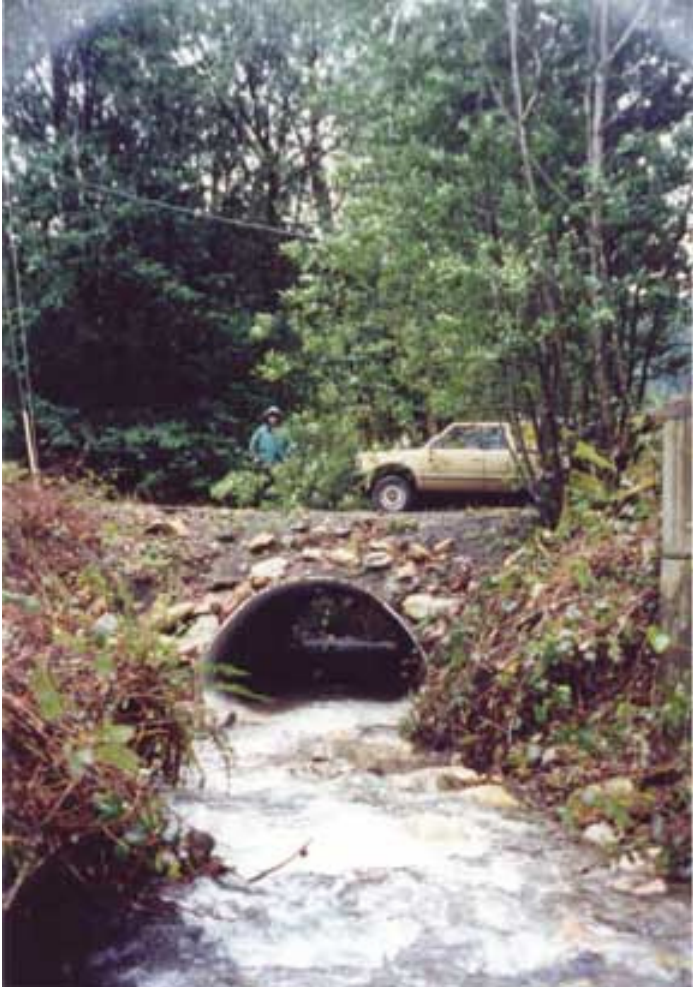
Looking downstream at the beveled inlet
