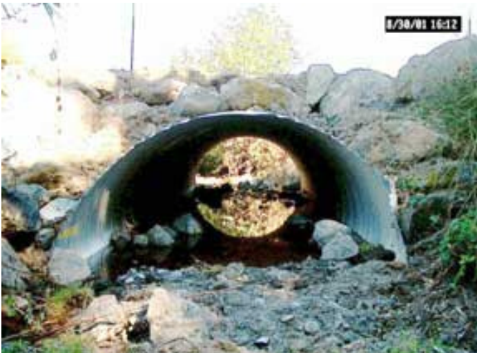
Inlet of downstream culvert following installation, 08
