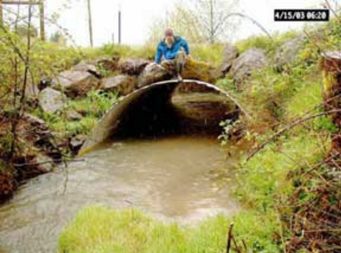
Inlet of the downstream countersunk culvert, 04/15/03
