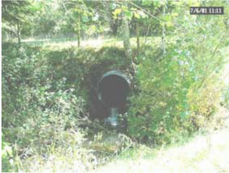
Looking at the outlet of the former culvert, upper crossing, 07/06/01
