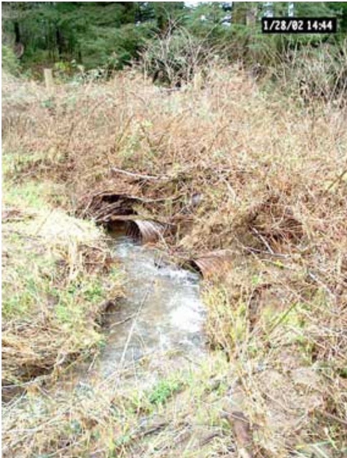
Looking at the former inlet of the lower crossing, 01/28/02
