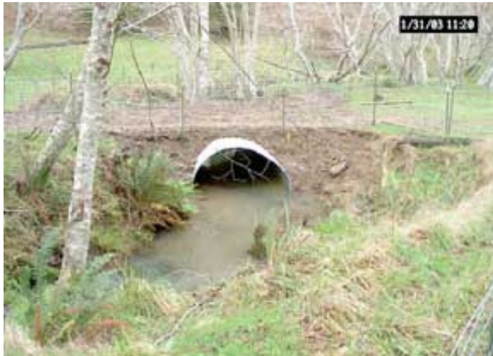
Looking downstream at the inlet following installation, 01/31/03
