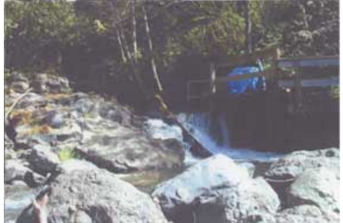
Side view of top jump over intake dam, 04/01
