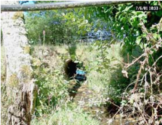
Looking at the former inlet of the lower crossing, 07/06/01
