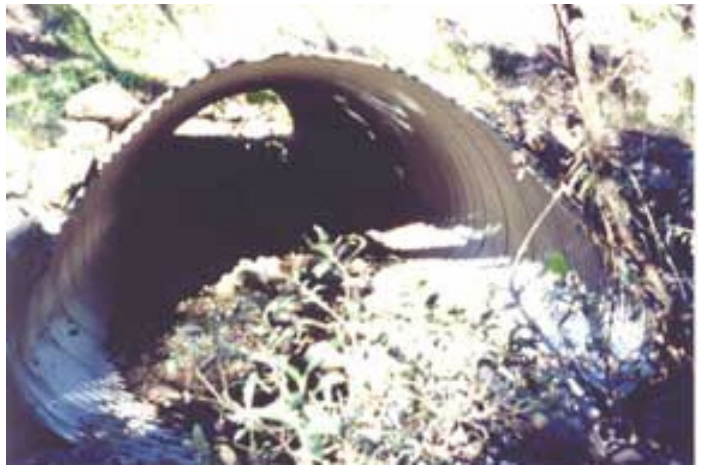
Looking upstream at headcut, where nick point migrated upstream. Looking downstream at mitered (beveled) inlet
