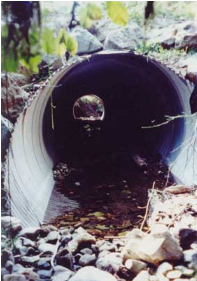
Looking downstream at the material collecting at the inlet, 09/30/99 Outlet, no drop, 09/30/99
