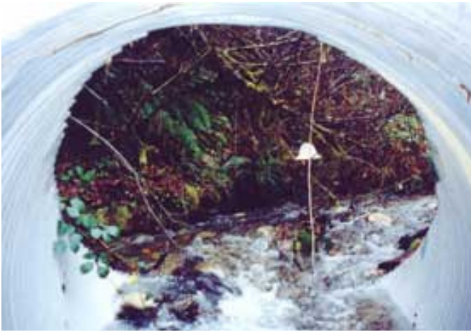
Looking upstream from inside the inlet, 01/12/00
